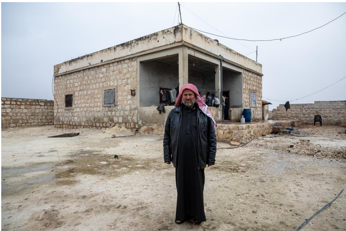
Abd Alhameed Alhashemi, whose family recently returned to southern Aleppo, stands in front of his home, which received UNHCR shelter repair interventions to ensure the doors and windows are sturdy enough to withstand the winter cold. © UNHCR/Hameed Maarouf
