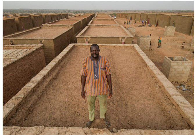
Adama Bamogo, an IDP in a UNHCR shelter in Kaya northern, poses on the roof of a Voute nubienne house.
