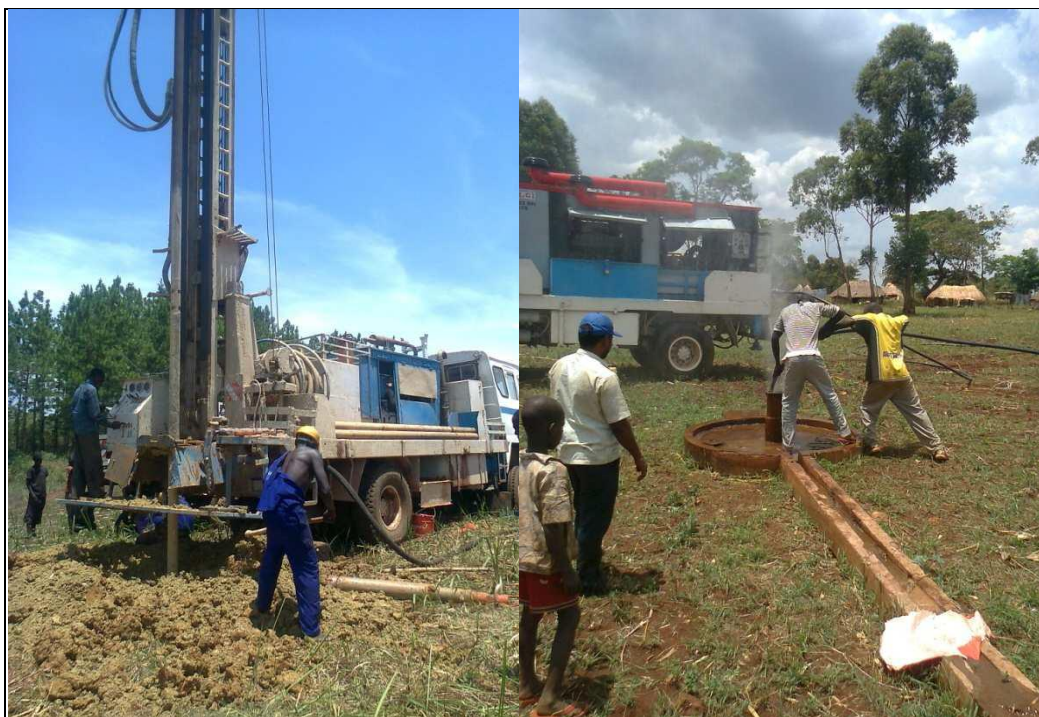
Borehole rehabilitation and drilling is ongoing in all three locations where South Sudanese have arrived. Here, workers in Kiryandongo refugee settlement labour to return a borehole to a functioning state. ©UNHCR / M. Njeru.
