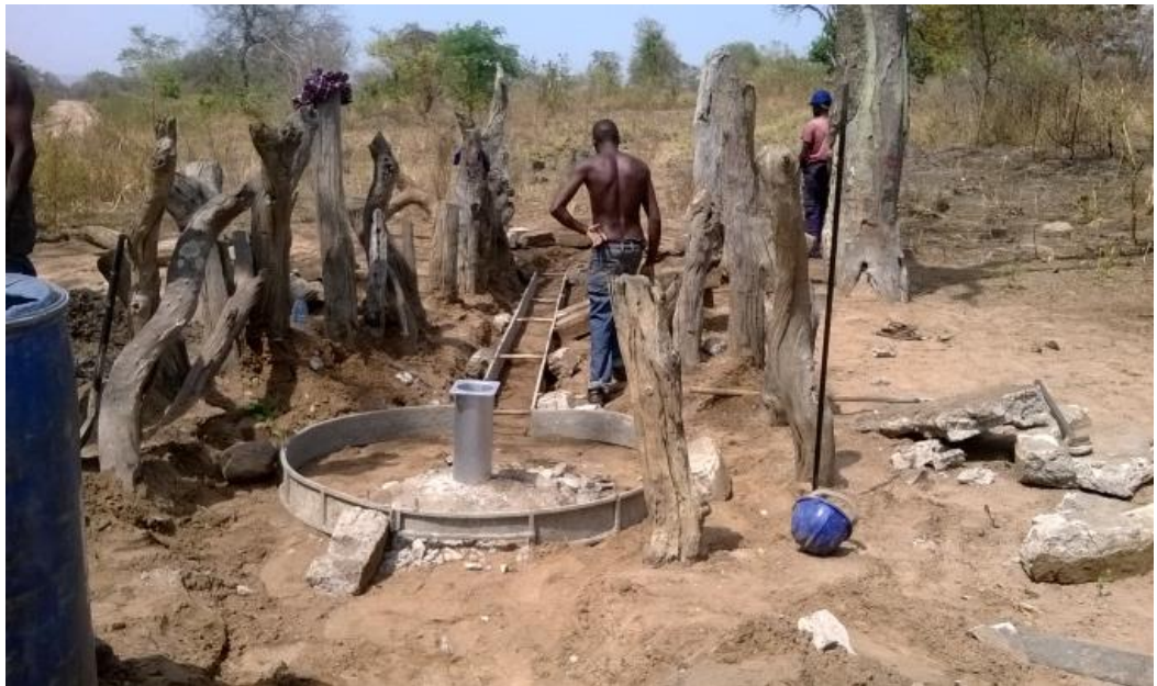
Borehole rehabilitation by ZOA Uganda in Rhino Camp, Arua. © UNHCR/A.Ndungu
