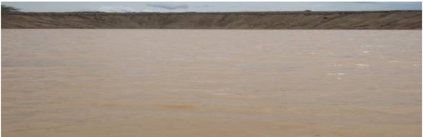
The Nakoros water pan is used for arid and semi arid lands (ASAL) irrigated farming, for livestock and for domestic use (using filters). It is expected to serve the community for up to five or six dry months every year.
