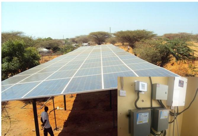
Photovoltaic modules and solar power inverter at a borehole in Hagadera
