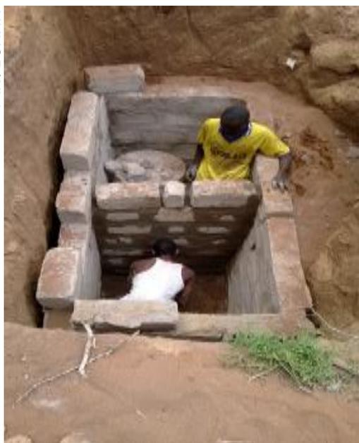
*Construction of a pilot twin pit latrine in Kambioos*
