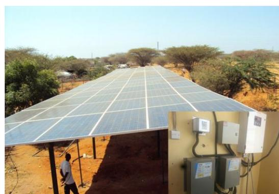
Photovoltaic modules and solar power inverter at borehole in Hagadera
