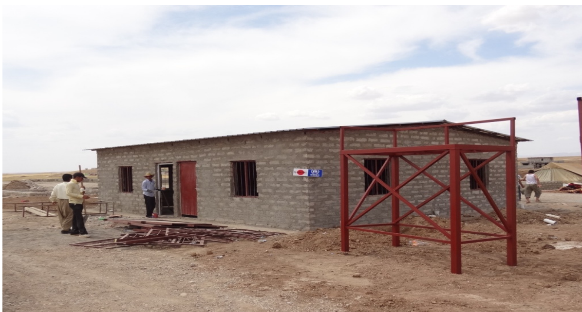
The communal kitchen for the singles in Domiz camp
