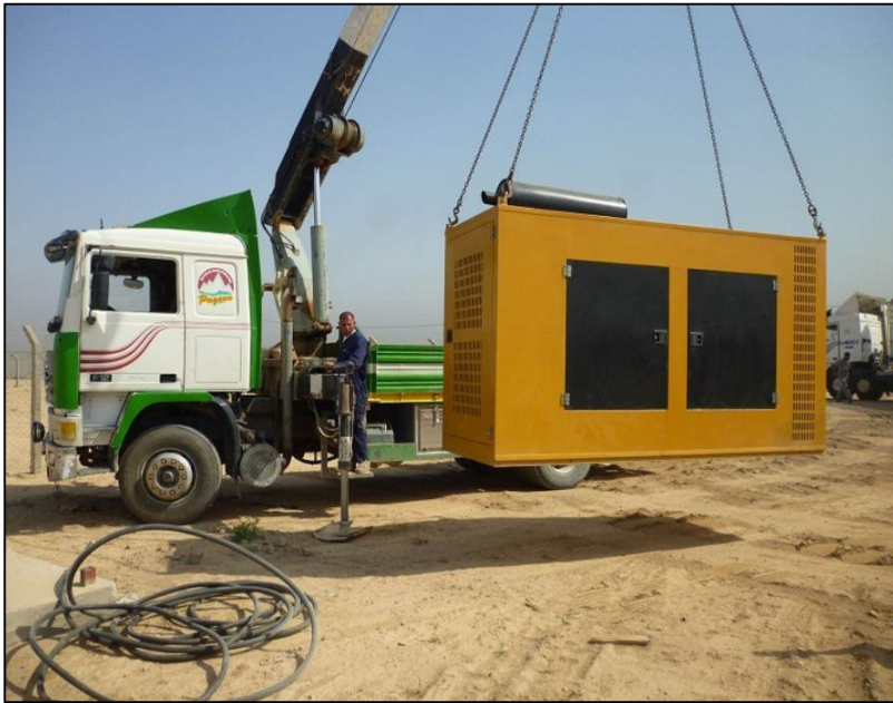
Installation of the generator in Camp 3 in Al Qa'im. IRW/Wissam
