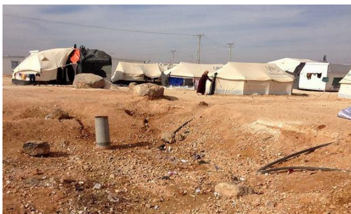
Photo 1: Underground WASH Centre tank with metal cleanout pipe showing above ground and small pipes connecting households to tank.
