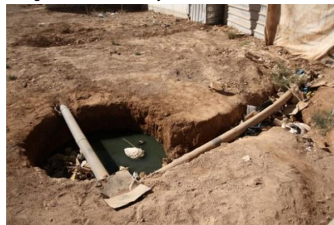
Photo 3: Underground connection pipes leading to wastewater pit.
