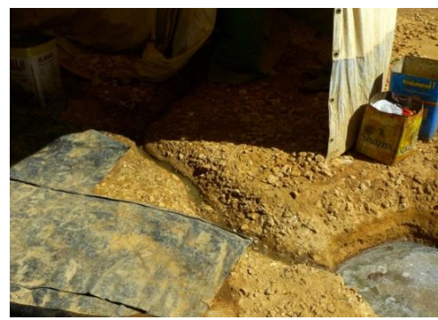
Photo 5b: Ditch leading wastewater from tent kitchen to outside pit.
