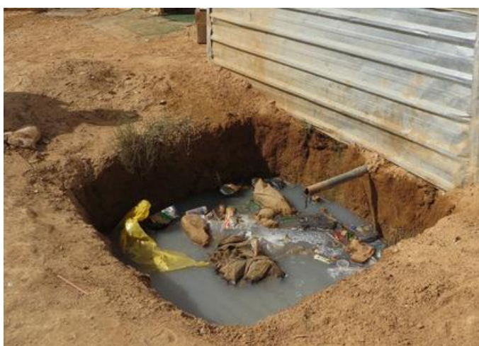
Photo 2: Wastewater pit with grey water inlet through pipe.
