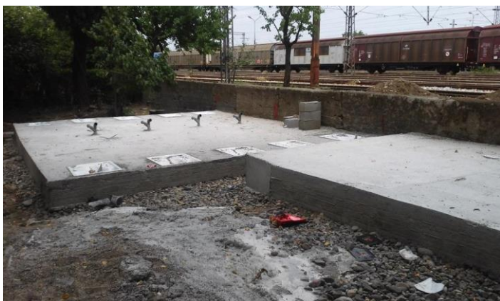
Gevgelija WASH facilities progress on August 6 th
