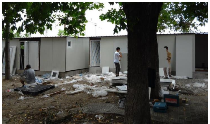
Gevgelija WASH facilities progress on August 11 th
