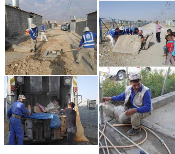
WASH service provision, operation and maintenance in on Arbat Camp, Sulaymaniyah, UNHCR and ThW. Clockwise from top left: Installation of manholes; replacement of manhole covers; repair of household water connections and garbage collection.
