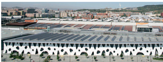
Figure 8. Medium scale grid-tied rooftop system (source: ICAEN [3])
