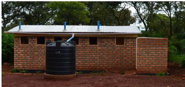
Newly constructed school latrines in Mtendeli Camp. @UNHCR/Sadick Mohamed
