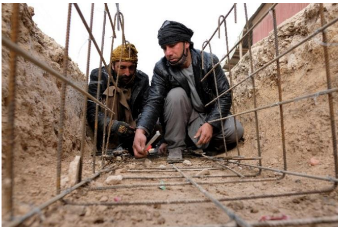
Returnees construct anti-flood canal as part of community based protection cash-for-work initiative to support community assets and infrastructure in Kabul province. ©UNHCR/ S. Rich
