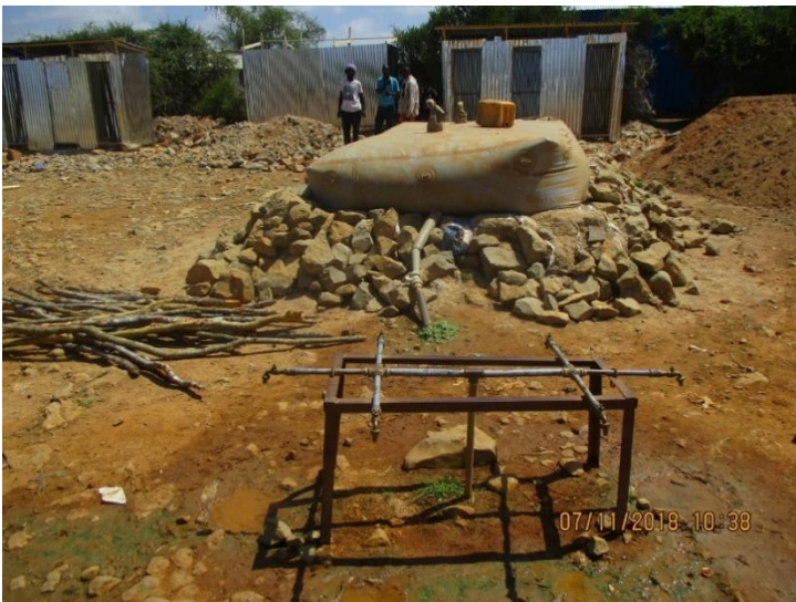
Water bladder at Guudka for immediate delivery of safe drinking water to IDPs without water sources
