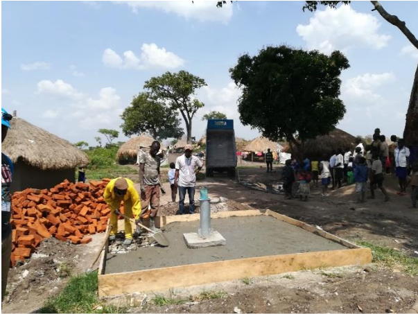
Borehole construction at Biringi settlement © UNHCR/Lopes
