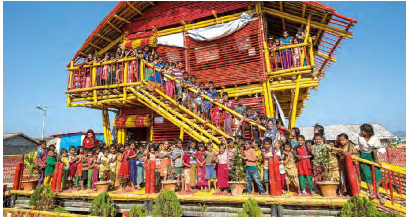
Sunflower Learning Centre in Kutupalong Extension Camp 4, Bangladesh, is the first two-storey building in the camp and was designed to save space and reduce overcrowding.
