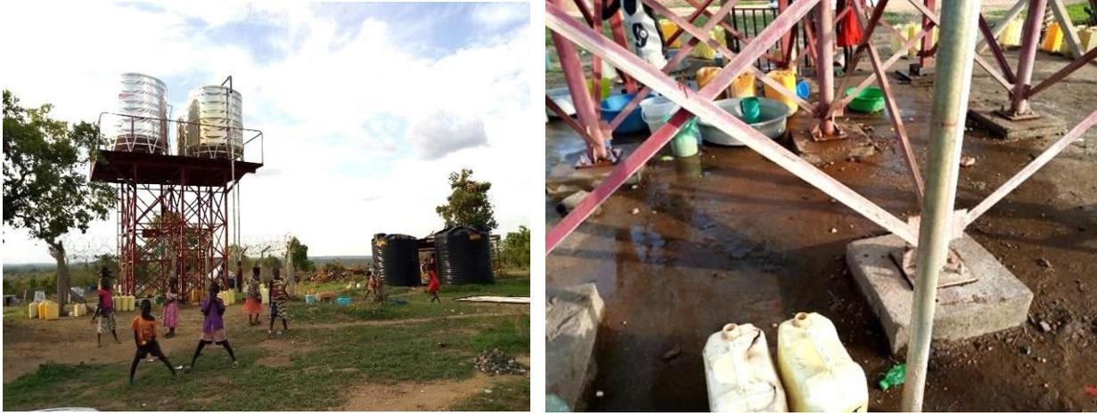
*Figure 6-4: Water spillage at a storage tank in Rhino Camp Settlement.*
