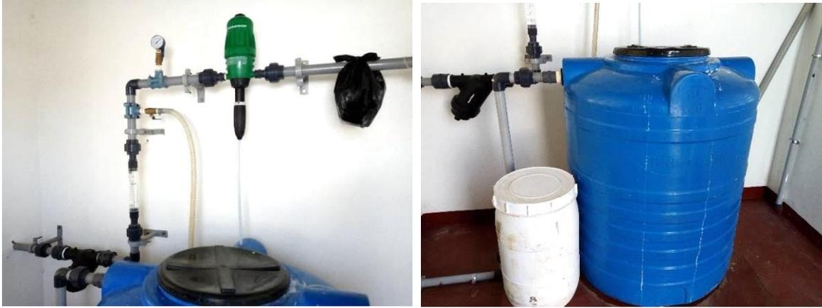
*Figure 6-5: L-R Online chlorine dozer, Chlorine drum next to mixing tank. In case of chemical spillage and or fumes the corrosive chemical may attack the electrical control panel housed in same house.*
