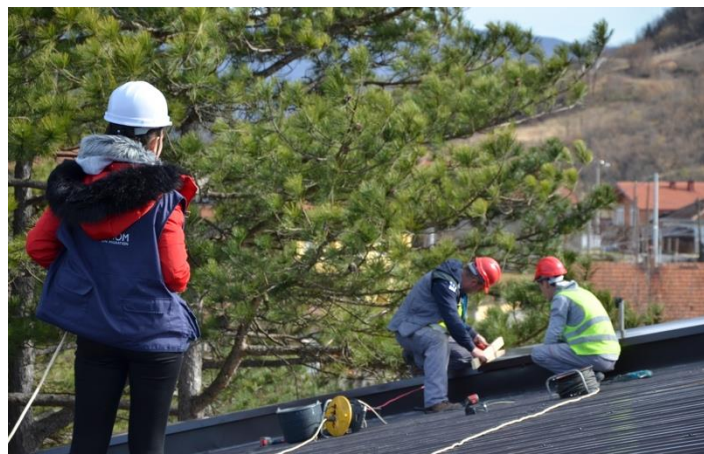
Repairing the roof in TRC Borici, IOM
