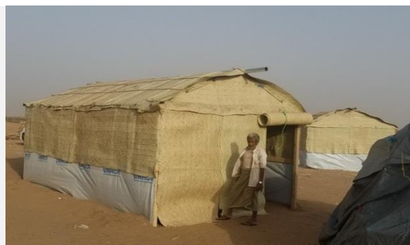
A Tehama is a type of an ESK, with an extra layer of palm leaves (Khazaf) produced by IDPs and host community members. This shelter is
