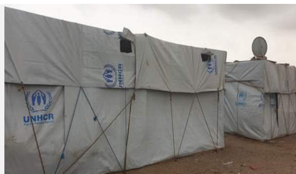
An Emergency Shelter Kit (ESK) is the UNHCR standardised shelter that consists of plastic tarpaulin sheets and sisal ropes. These last up to
