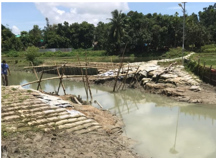
A burst dam in Nayapara refugee camp (Teknaf) which has been recently damaged by a surge in heavy rain. Photo: UNHCR
