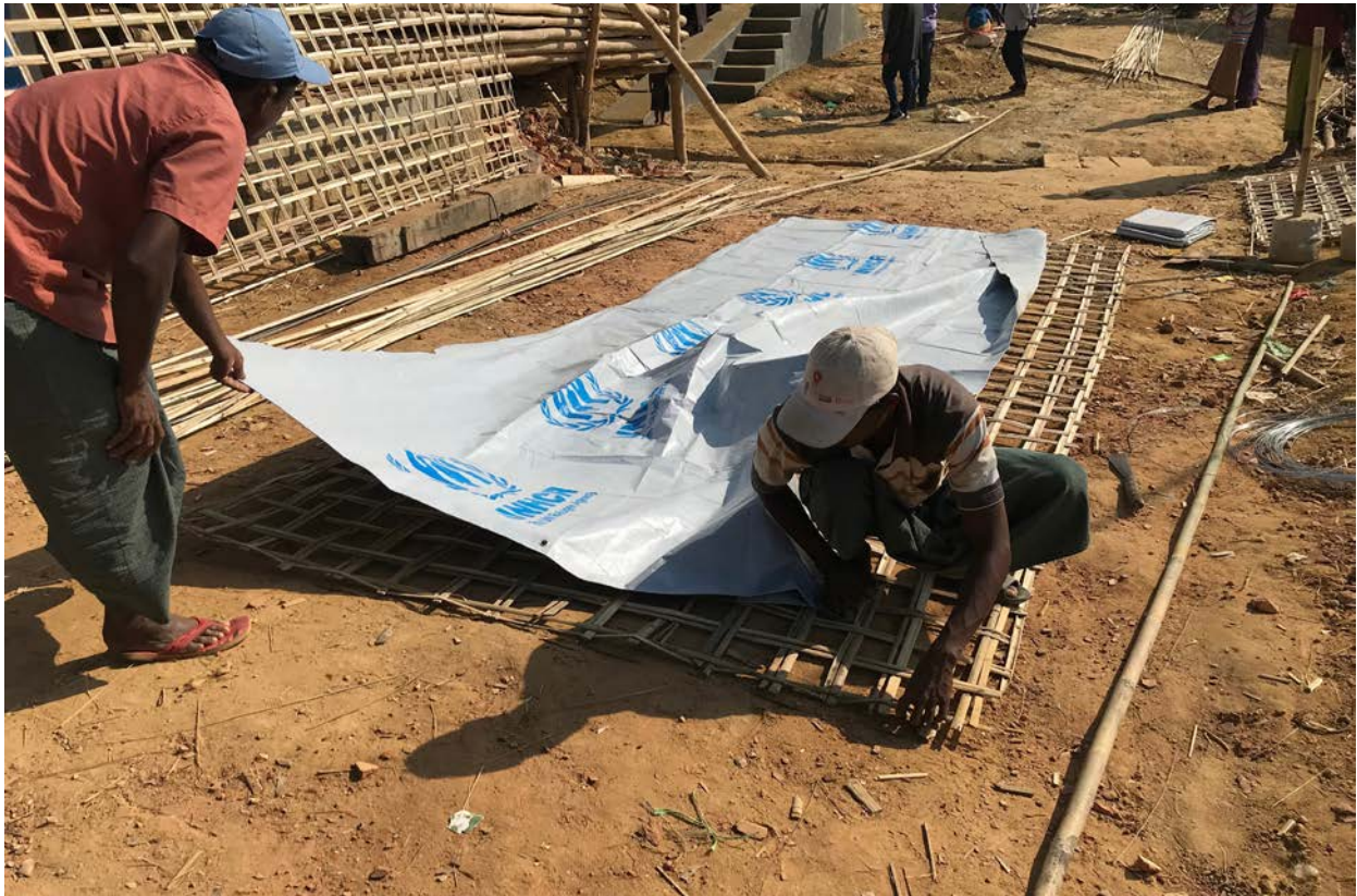
Bamboo and Tarpaulin are being used to build shelter © UNHCR
