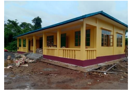
School construction in Kayin State, Photo UNHCR
