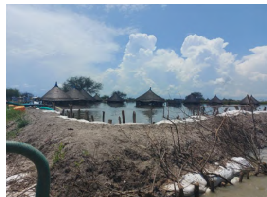
Flood-affected houses in Twic East. Photo: DRC.
