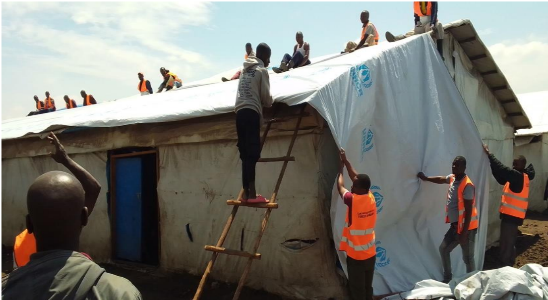
Repair of leaking roofs at Nyakabande Holding Area. Photo ©CAFOMI
