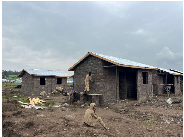
Shelter construction in Alemwach site, Amhara region ©UNHCR
