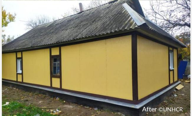
The repair and insulation work for a house damaged by conflict is finished in Kyivska oblast through UNHCR's shelter programme. Before the repairs, the wooden house was vulnerable to the cold and expensive to heat. With the new layer of wall insulation, the house is able to warm the family.
