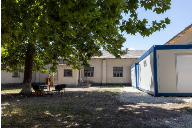
Rural RAC exterior
