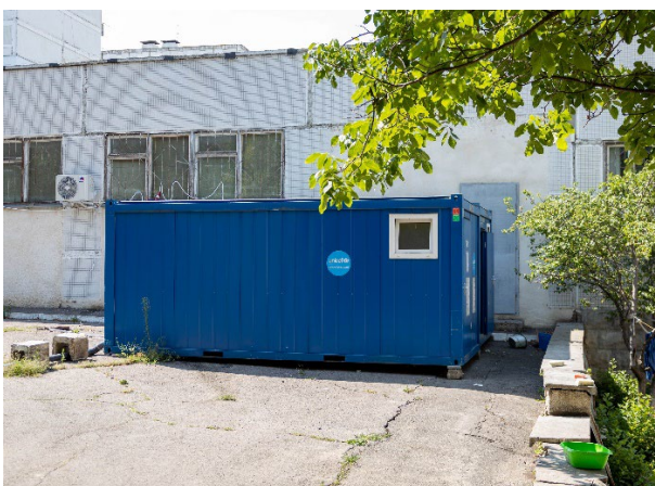
Outdoor sanitation block at a Chişinău RAC Photo credit: Lottie Stevenson/Oxfam
