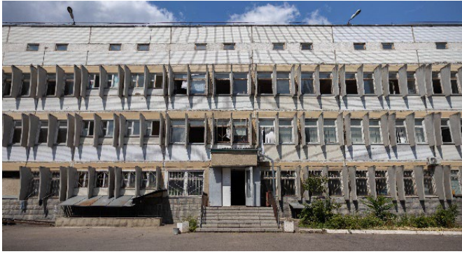
Chişinău RAC exterior
