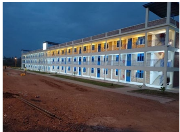
The completed Ground+2 Refugee Apartment with the capacity to host 360 persons which opened in xxx. Since its opening the capacity of the ETM increased to 700. © UNHCR
