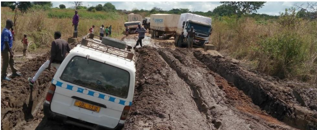
Road conditions in Rhino Camp settlement. @UNHCR
