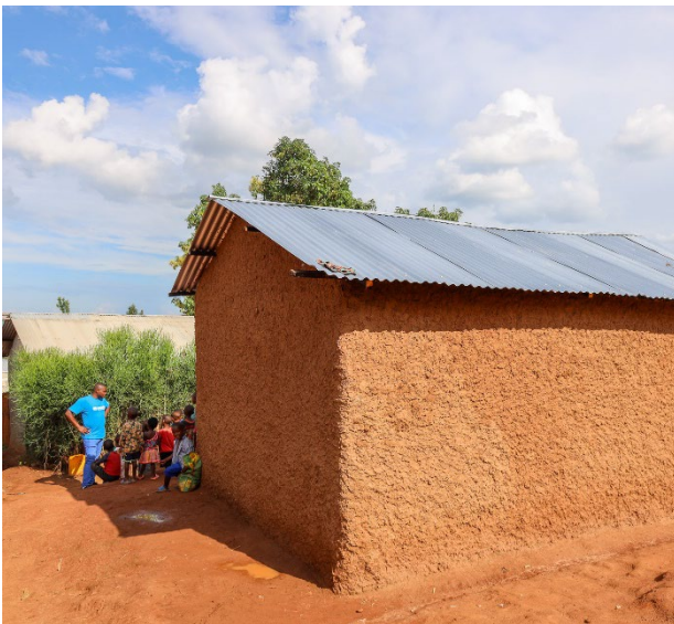
A new shelter is constructed in Nyabiheke refugee camp.
