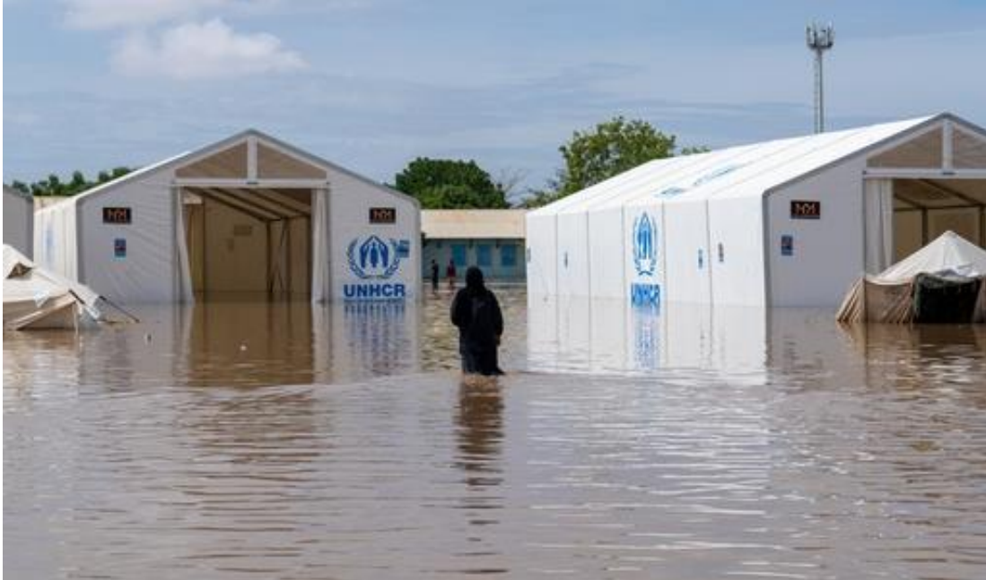
UNHCR Rubbhalls in Omar Ahi Musa gathering site, Kassala town which were used as temporary shelter and were accommodating some 8,000 people were flooded by the rains. © UNHCR
