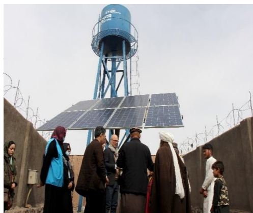
Construction of water well for 250 HHs in Kahdistan of Injil in 2022 @UNHCR
