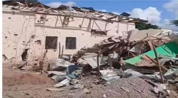
Figure 2: The University of Southern Somalia damaged by the conflict
