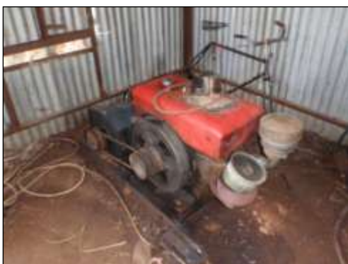
Pumping station old / 10 KVA generator to be replaced
