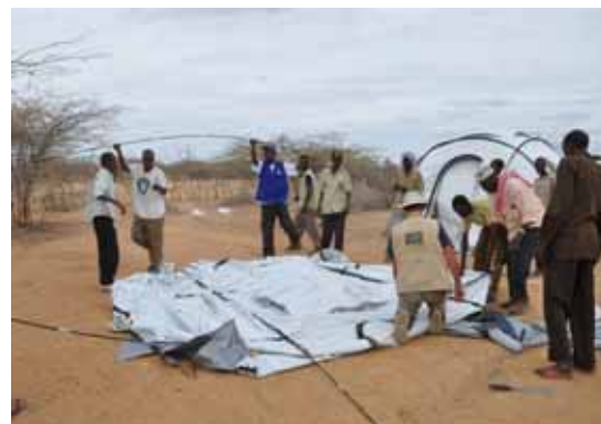
Set up of emergency shelters in the Ifo extension (Photo IOM©)
