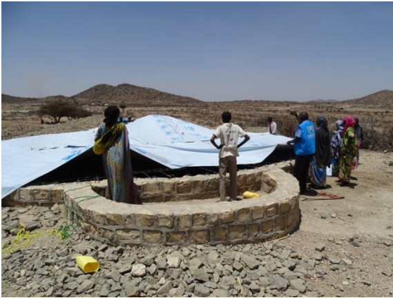
UNHCR staff installing plastic sheet cover over a water storage Berkerd (circular concrete underground tank) in the drought affected area in Goroyocawl village near Borama, Somaliland, . ©UNHCR/ F. Andi - March 2016
