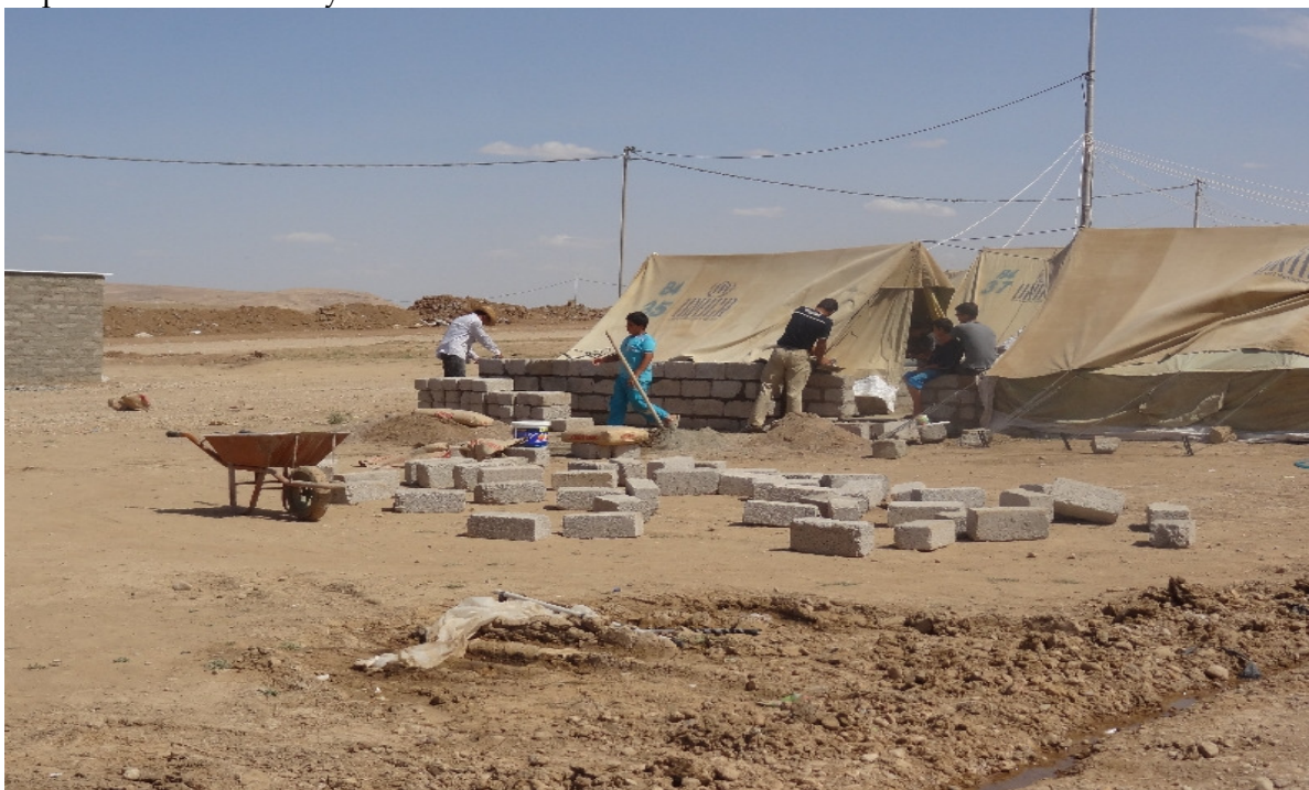
Constructing of walls surrounding the tents
