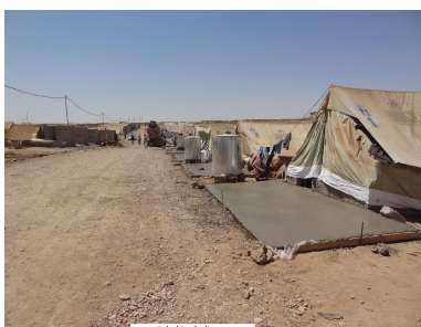
Casting foundations of cooking area
