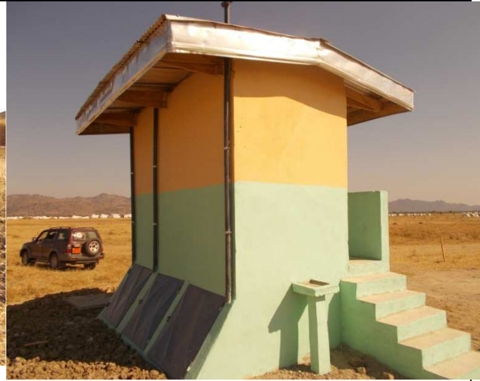
Latrine ECOSAN - IEDA (infrastructures scolaires)
