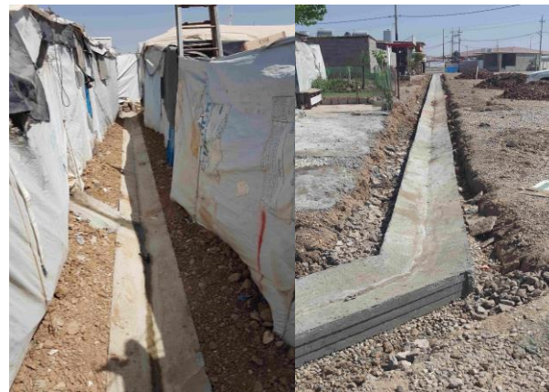
Construction of new open drainage channels behind shelters and along roadsides in Domiz 1 camp, Duhok. UNHCR/Iraq/2016
