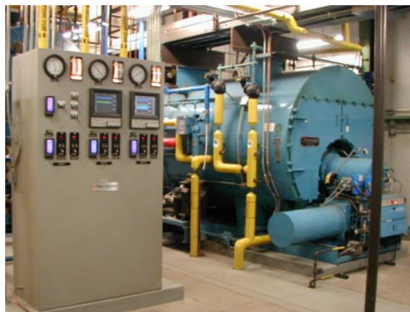
Figure 26: Hays Cleveland's O<sub>2</sub> trim system installed on two boilers
