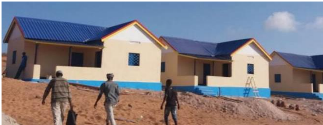
Newly constructed shelters in Kismayo. © ARC / Kismayo, October 2017
