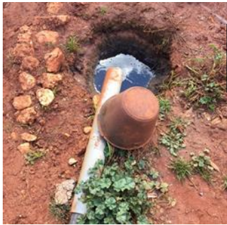
Figure 5: Greywater soakaway pit and bucket for emptying, Bouday A
