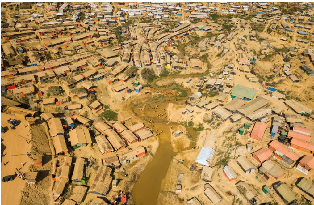
UNHCR is undertaking emergency preparedness works, including clearing and strengthening drainage channels, as part of the Site Maintenance Engineering Project (SMEP), a joint initiative of UNHCR, IOM and WFP. © UNHCR/Roger Arnold
