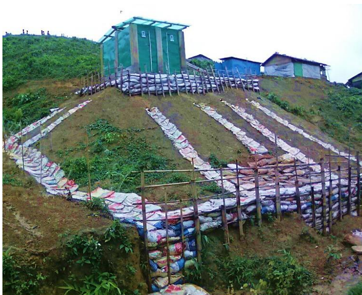
UNHCR piloted soil erosion mitigation measures around WASH facilities in Camp 5, Kutupalong settlement. © UNHCR/ T. Teh
