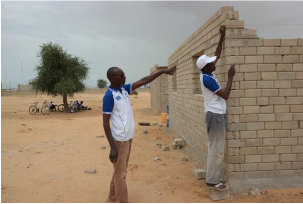
Examples of two construction techniques – Traditional “construction sans bois” (Chetimari – houses 18m 2 ) and “Hydraform Construction” (Diffa Town – houses 24.5m 2 ). Both techniques are adapted to the context and sensitive to the environment (UNHCR).
