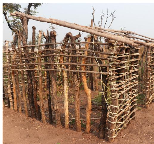
Figure 7: The side of a timber pole home in Lóvua settlement ©UNHCR/Omotola Akindipe
