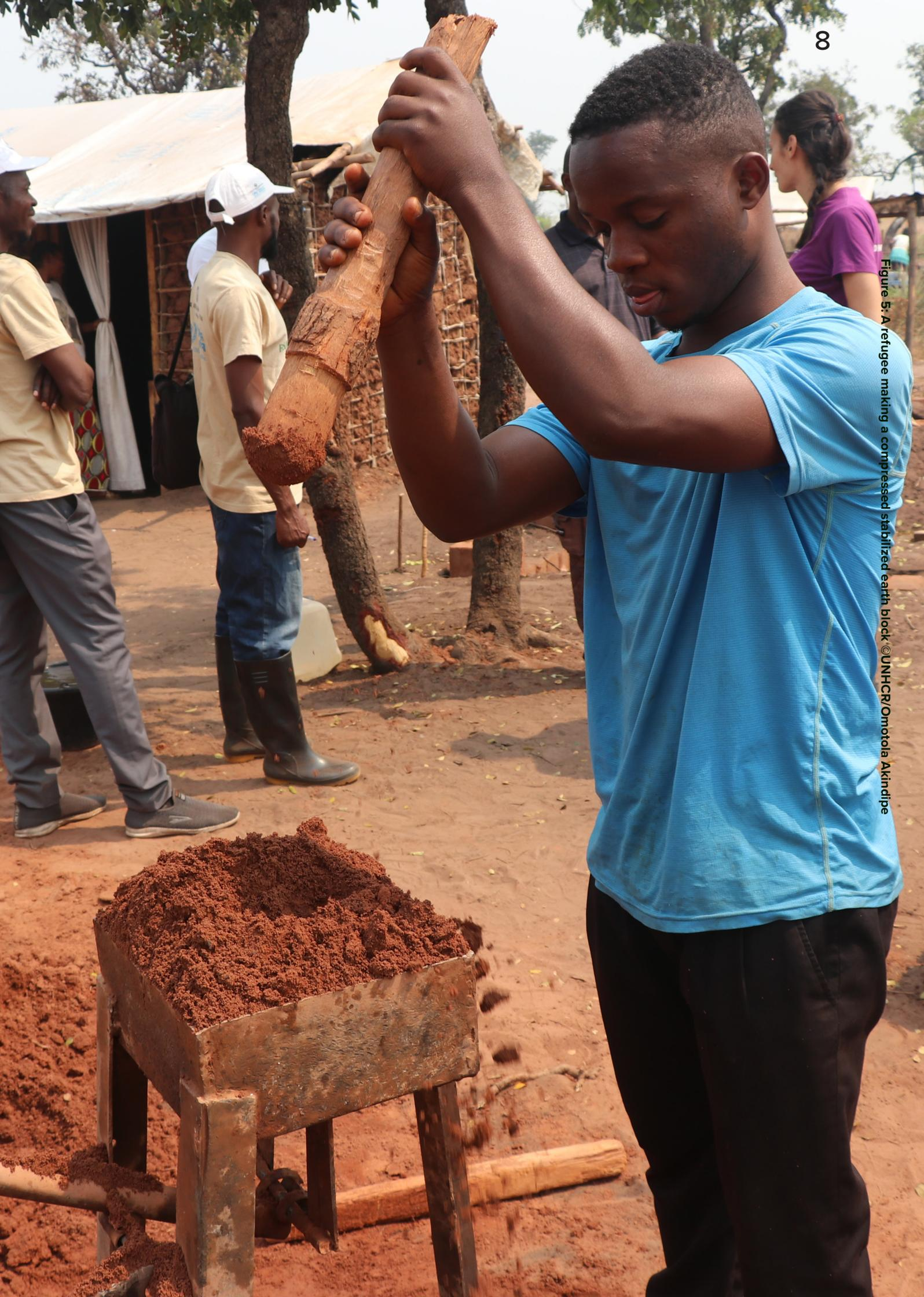
Figure 5: A refugee making a compressed stabilized earth block © UNHCR/Omotola Akindipe
